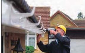
From outlet, fix support brackets at a maximum of one metre centres.
