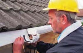
Insert gutter to the 'insert to here' line on the first fitting. At the other end of the gutter mark the position of the next fitting on the fascia.
