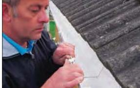
Fit length of gutter and stopend, with support bracket at furthest end.
