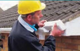
Fit top offset bend to outlet, then using bottom offset determine length of pipe required.
