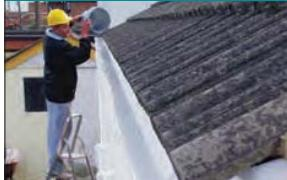
Check water tightness by blocking off any outlet and performing a static water test.
