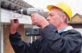
Fix support bracket at furthest end and run a string-line to the outlet.
