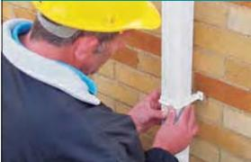
Fit a pipe clip below the bottom offset, then at a maximum of two metres apart.
