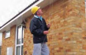
Before starting work, identify position of drain, run a plumb-line and fix gutter outlet. Check fascia is level and determine fall (if required).
