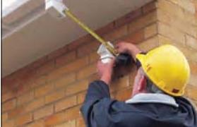
Remove gutter and fix next fitting using your mark line. Ensuring fittings are level by using a string line.
